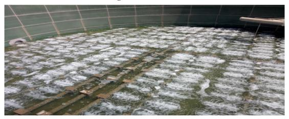
SBR Under Testing for Proper Mixing
