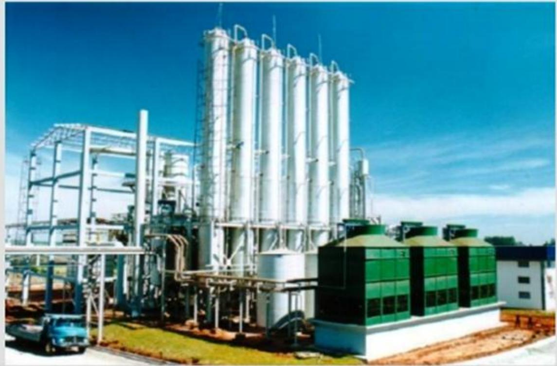
**SODIUM BICARBONATE PRODUCTION PLANT – NaHCO<sub>3</sub> – INTEGRATED TO AN ETHANOL MILL**
